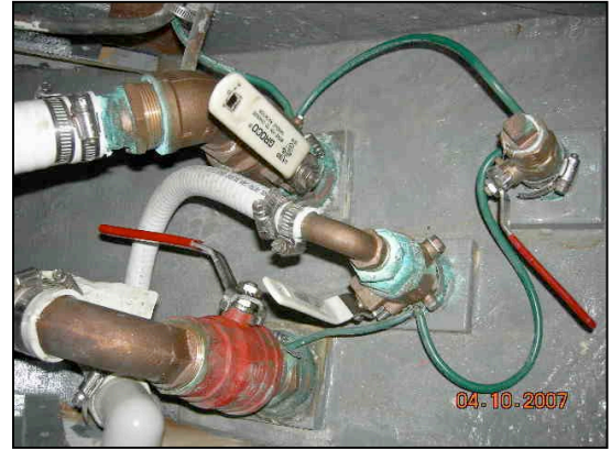
New sea valves, bonded
